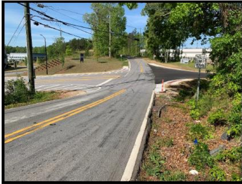
Photograph 1 – Factory Shoals Road Facing West at Douglas Hills Road
